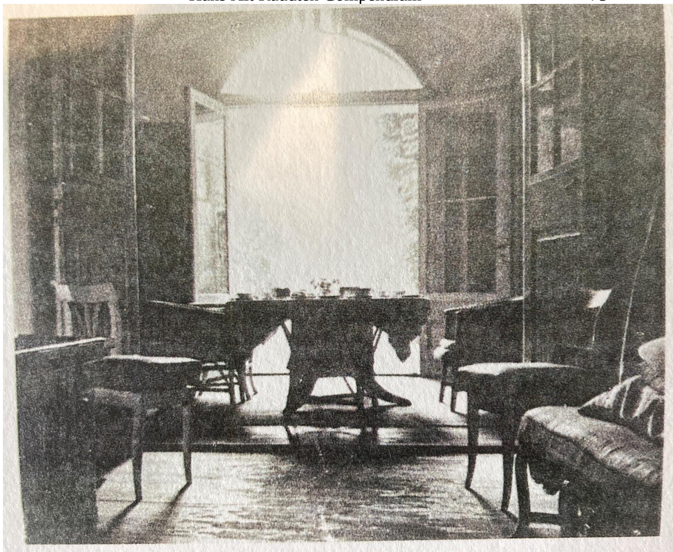
One of the ground floor rooms
