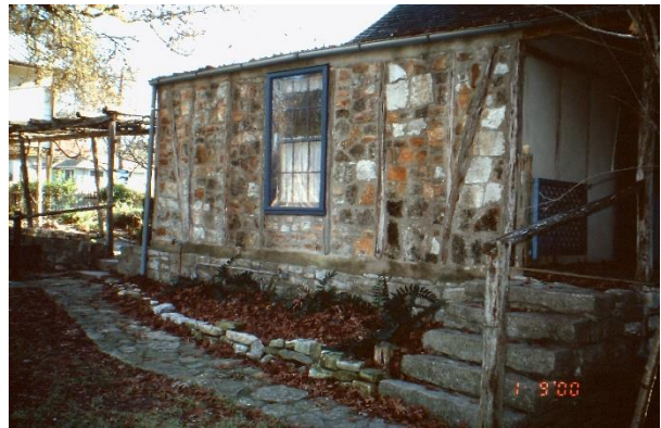
14d New Braunfels F Lindheimer house. Built in 1845 back view. The rear shows a Fachwerk (half timbered) skeleton filled with local limestone. Fachwerk is considered a typically German construction technique and was not given up until the mid 1860s when the Germans in Texas had figured out
