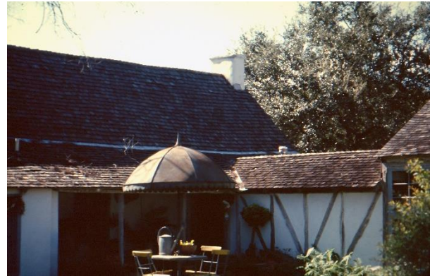
21m Castroville Peter Pingenot House Cabin and house connected with Fachwerk hall
