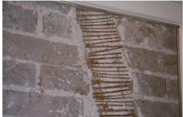
16d New Braunfels Lindheimer house stone wall with wood insert
