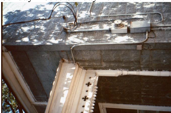
23b Fredericksburg. Christian Vogel Sunday House. 418 W Austin Street or is it 409 W San Antonio Street. Built late 1800's. This house is an example of the popularity of covering a wooden house with embossed tin to resemble stone. This embossing was done in
