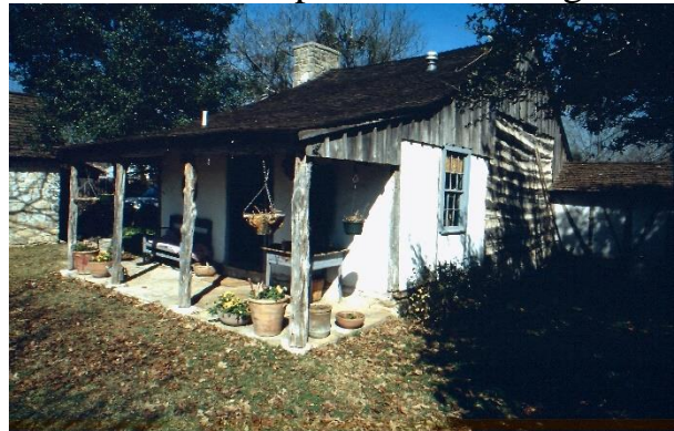
05L Castroville Peter Pingenot House. Log cabin added to house for more space. Cabin over cellar.
