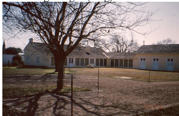
18M Castroville Bippert-Kueck House Example of Oldenburg Langes (long) House. Bippert built a picket structure in 1847 with one room 7 1/2 ft wide and 21 ft long home with a dirt floor. Roof was first thatched and later shingles. Heinrich Kueck from Aurich,
