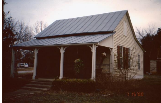
15f or 11g Comfort Otto Brinkmann cottage 602 (or 701) High Street. Built 1860 for Otto and brother, "Bachelor Bude". Timber frame (Fachwerk) filled with native stone, a technique introduced in Texas by German immigrants.
