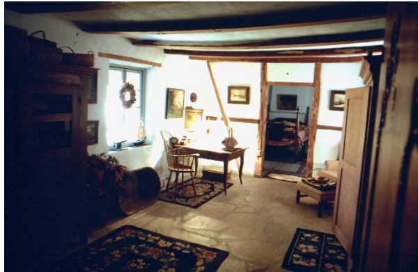
09L Castroville Pingenot cabin inside with timbers "Fachwerk"
