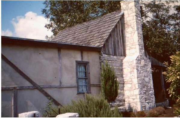
05a Fredericksburg. Kammlah family home and store. 325 W Main Street. Built 1849. On grounds of Pioneer Museum. House outer and inner wall made of Fachwerk. It is believed, that they first dug the cellar and lived in it while they built their home.
