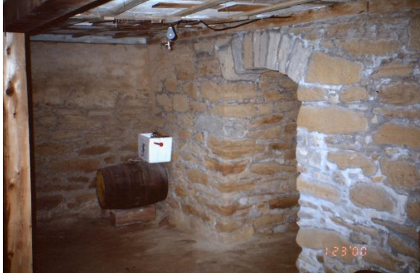
21f Shelby. Witte-Schmid House basement 1857 called "Das Haus". The cellar, with 20 ft walls of rock and wooden beams, was used for butchering. The wooden ceiling laths are filled with straw and plaster for insulation.
