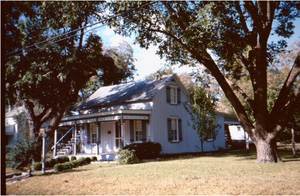
10b Fredericksburg Robert Jenschke House, 406 W Travis Street. Built in 1871 with board and batten frame construction. Later covered with embossed tin, Gingerbread trim, and turned posts. The tin made it look like stone, but has been removed by now. Outside stairway leads to loft. This type of house is commonly called a Sunday House because of the outside stairway.
