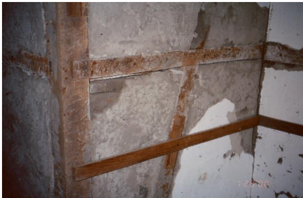
25f Shelby Witte-Schmid House 1857 called "Das Haus",. Upstairs fachwerk wall timbers filled in with adobe bricks.
