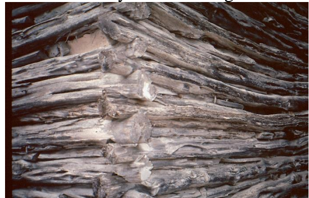
15c New Braunfels Conservation Plaza Welsch barn details. Log interlocked using V and saddle notches. Home style was Blockhütten.
