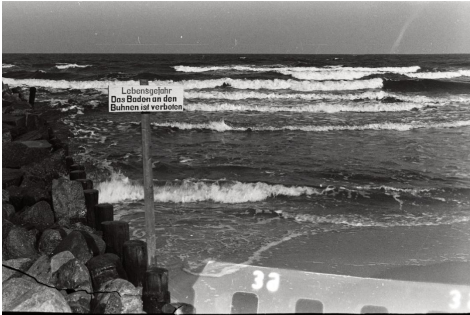
Lebensgefahr. Das Baden an den Buhnen ist verboten. Danger to life. Swimming at the groynes is forbidden. Groynes are low walls or sturdy barriers built out into the sea from a beach to check erosion and drifting
