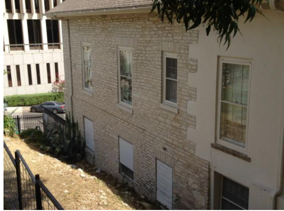
West side wall with difference in bricks from original structure to addition
