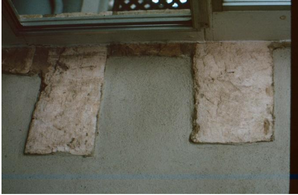
Difference in bricks and stones at junction of different sections of building
