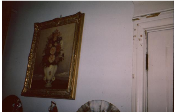
Termite damage to door jam
